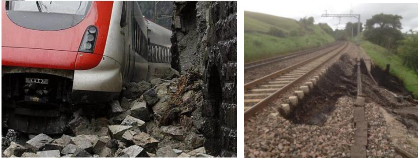
Figure 5. Dangerous situations on railway tracks: collapsed stones (left) and torn off super/substructure (right)
